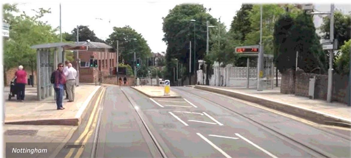
*Fig. 21 - Example of a narrow road tram stop. All traffic share, cyclists routed behind tram shelter*
