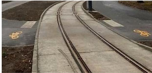
*Crossings not less than 45° should be engineered in at time of construction to ensure cycle safety*
