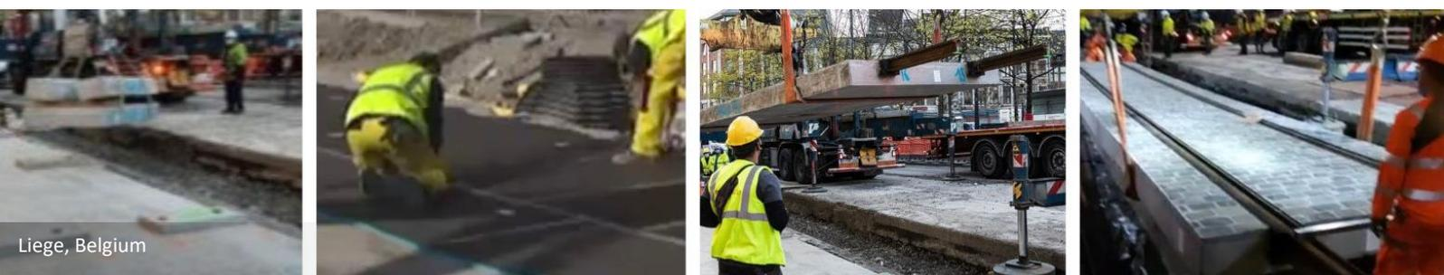
***Pre-formed track and pedestrian-friendly paving can simply be installed into a shallow trench on a "concrete float"***
