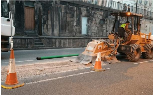
*It is possible to cut one tram-track at a time for minimal traffic disrupting and no diversion of services. Photo: pipe-laying in Bath*
